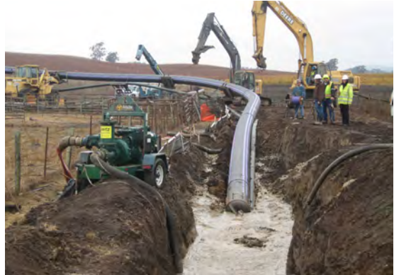
McMillen Jacobs Associates (then as Jacobs Associates) performed the geotechnical investigation for the Stanly Ranch HDD project, which involved crossing railroad tracks, the Napa River, and wetlands.
